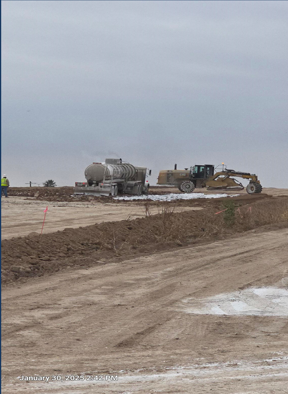
Lime placement in base at Jackson (FM2061)
